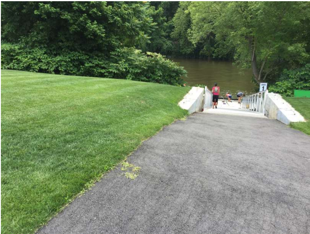
Completed Gangway Installation
