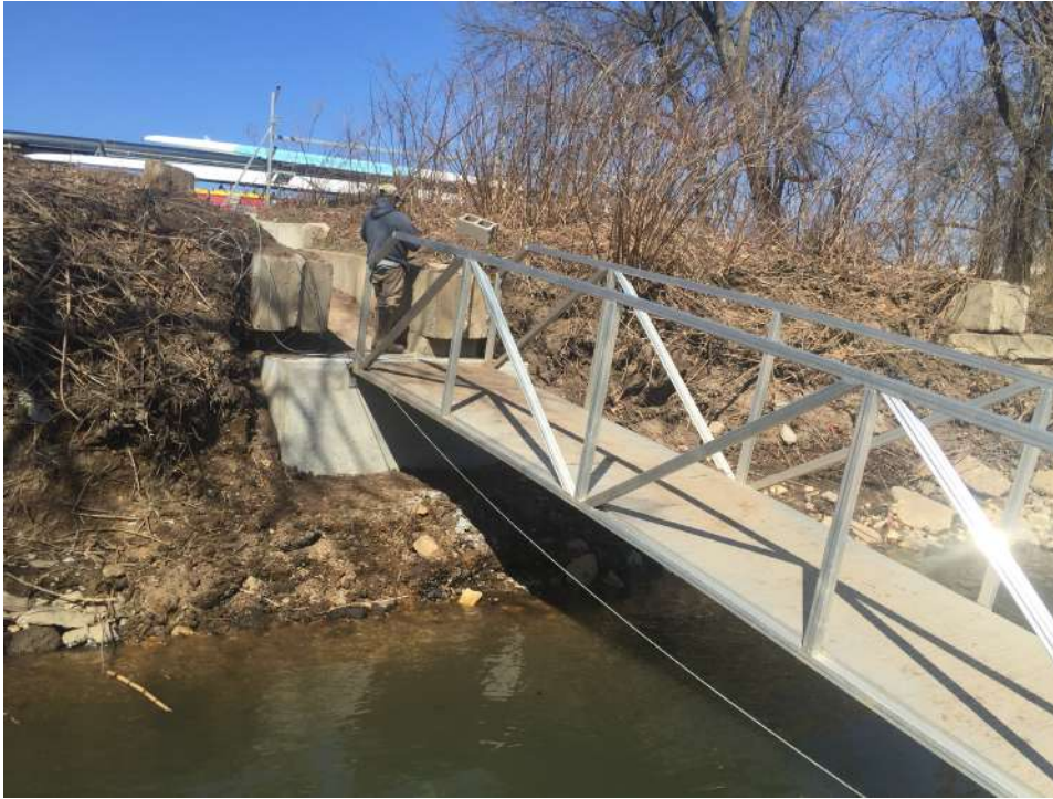
Gangway Reinstalled to new concrete bulkhead
