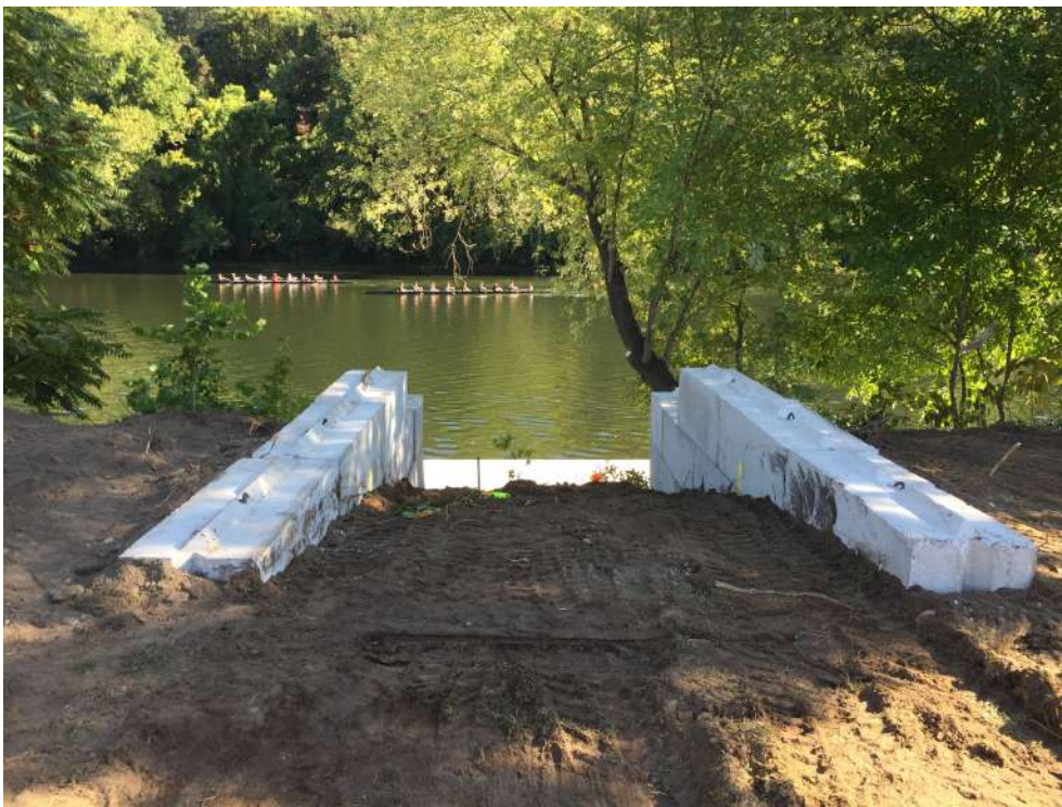
Excavation of new ramp and installation of concrete retaining walls
