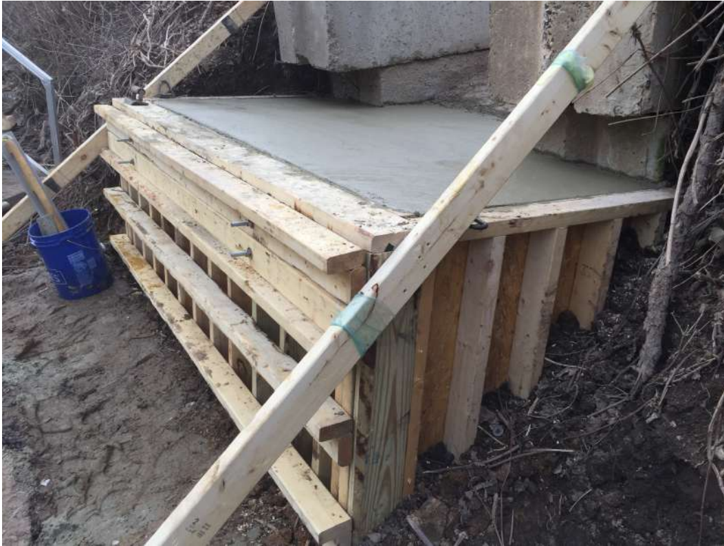
Newly Poured Concrete Bulkhead
