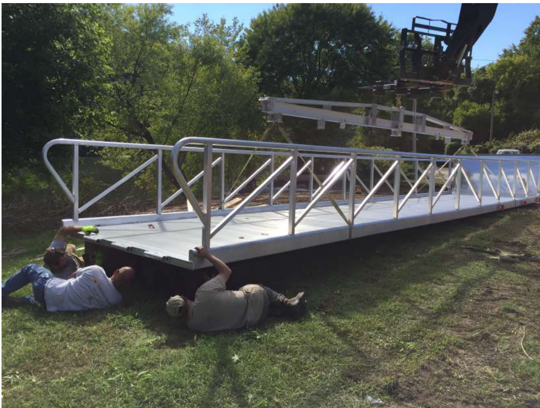
Supplemental Flotation being installed at bottom of BoardSafe HD Gangway
