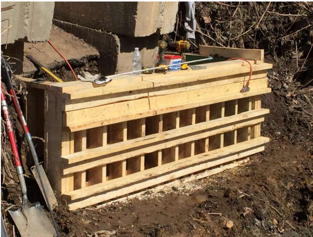
New Concrete Bulkhead being formed for Gangway attachment
