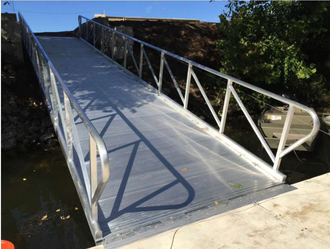
BoardSafe HD Gangway attached to existing docks
