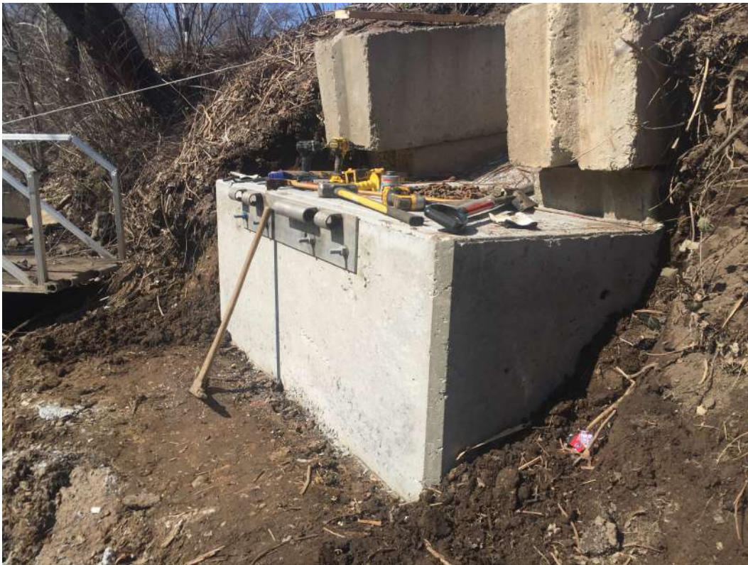
Newly Poured Concrete Bulkhead
