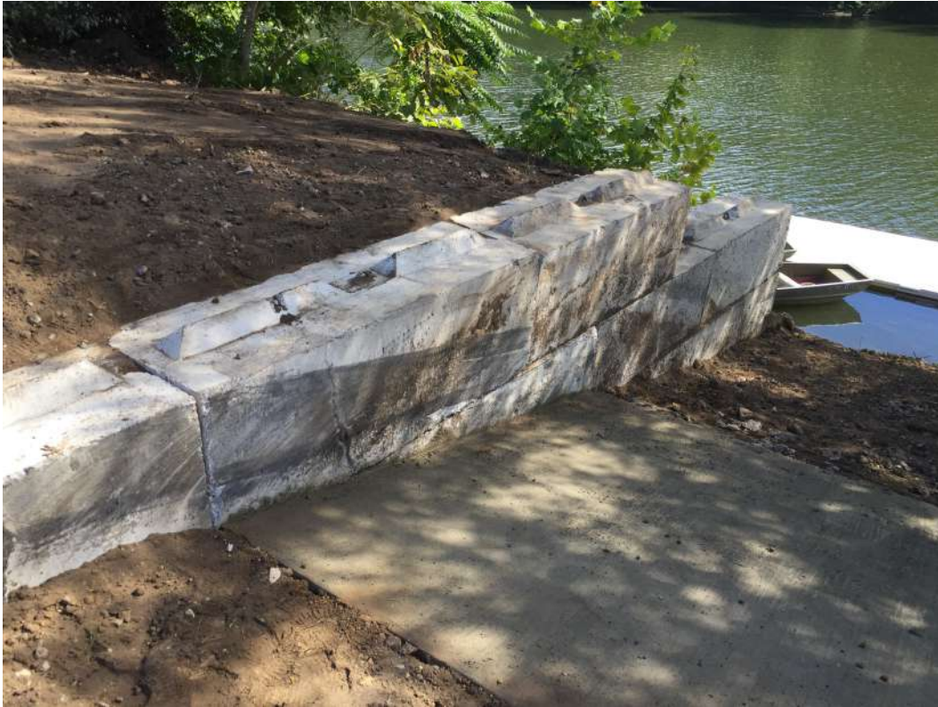
Installation of concrete landing for BoardSafe HD Gangway
