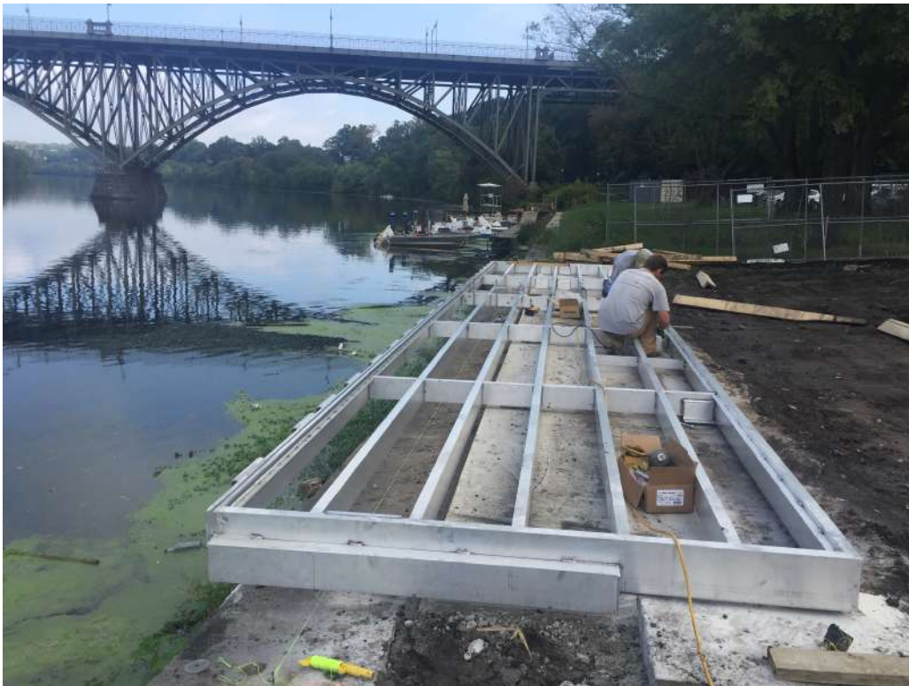
Cantilevered Deck installed on foundation system
