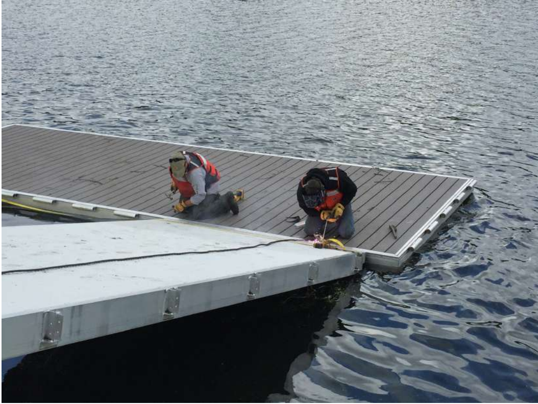
Installation of floating dock to gangway
