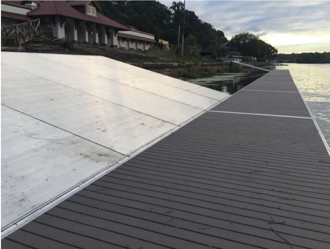
Day 1- Installation of floating docks and both gangways
