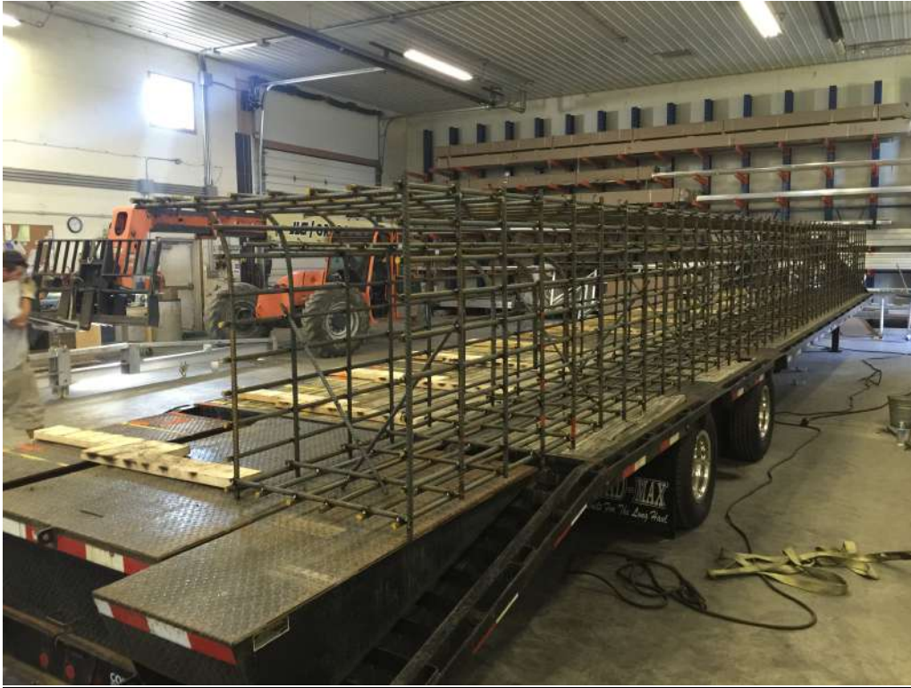
Rebar Cage being manufactured
