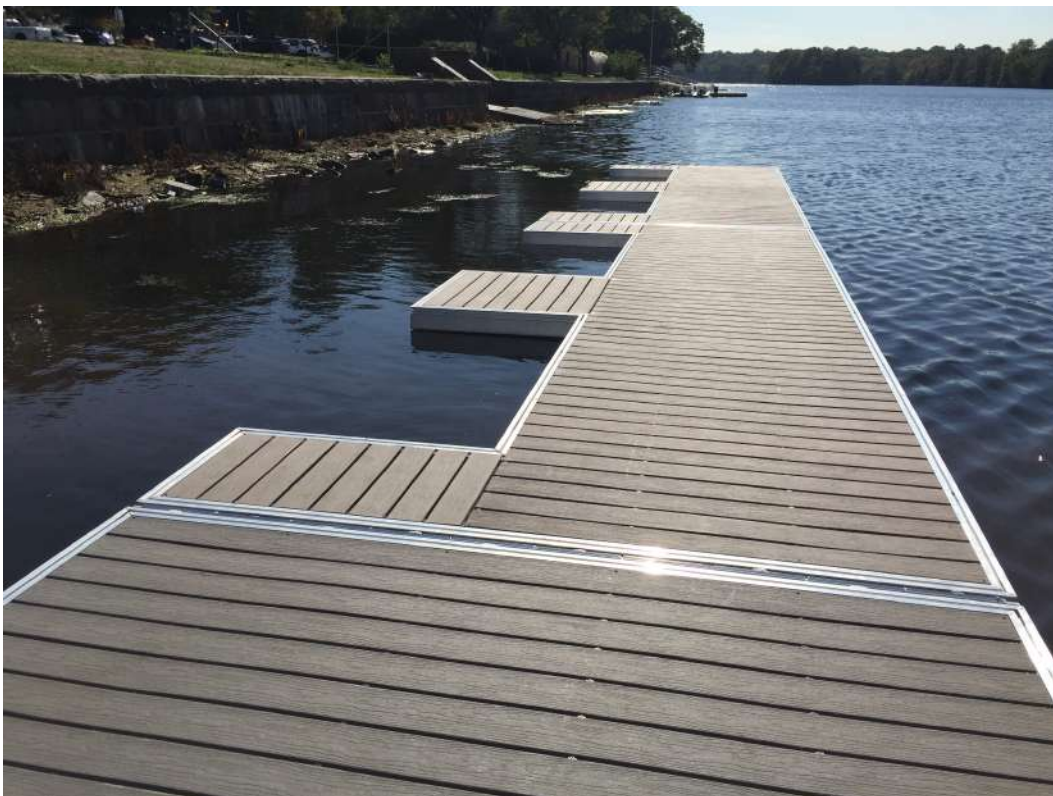
Completion of floating dock installation
