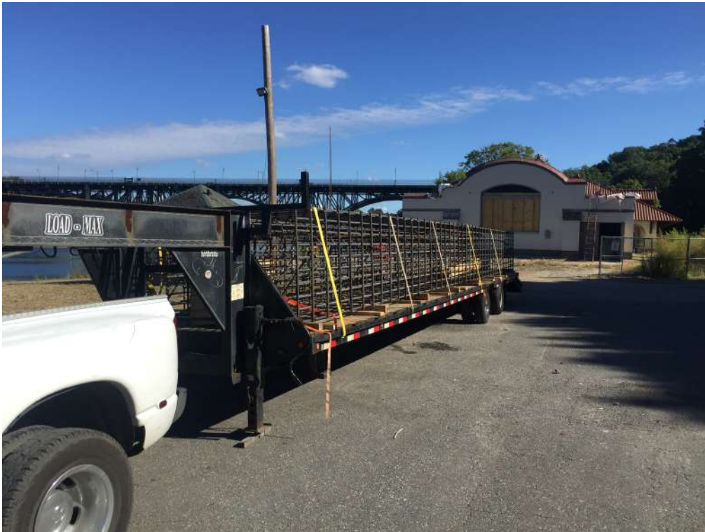
Rebar Cages delivered to job site
