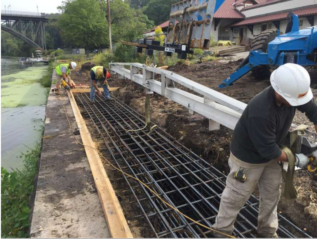
Rebar Cage being installed in excavated foundation
