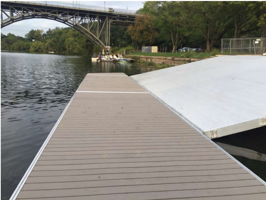
Completion of upstream gangway
