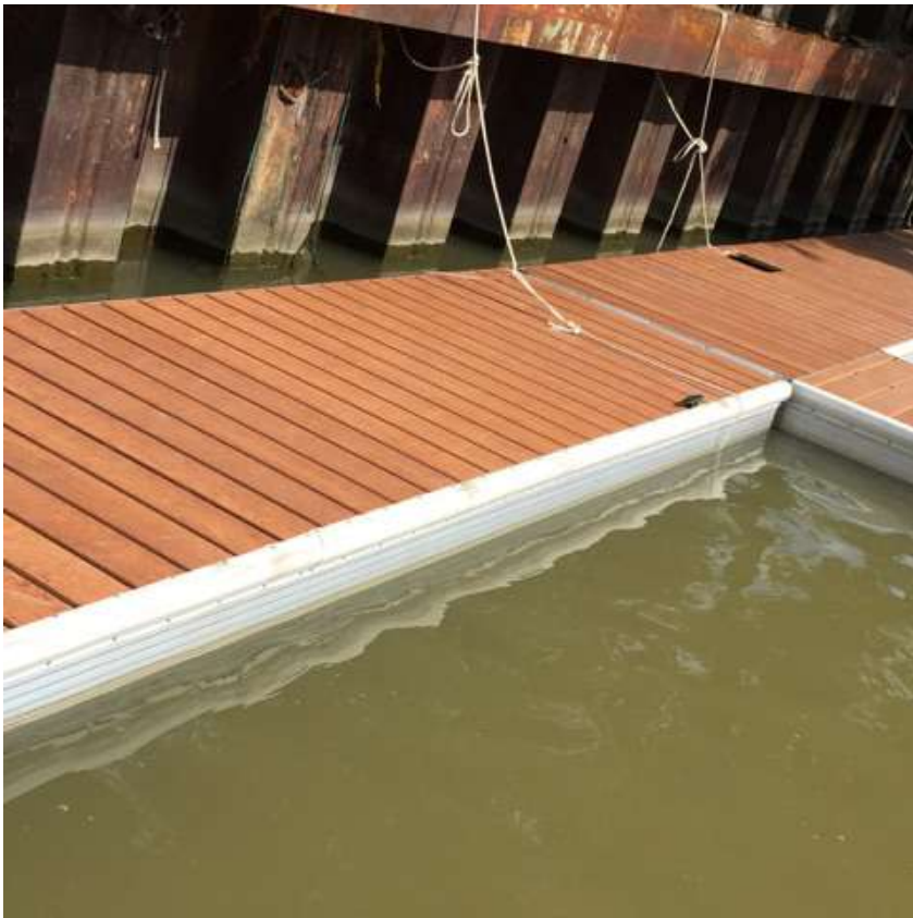
BoardSafe 50 Series Low Profile Docks being installed
