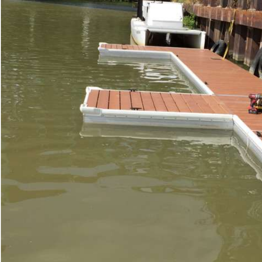
BoardSafe 50 Series Low Profile Docks being installed
