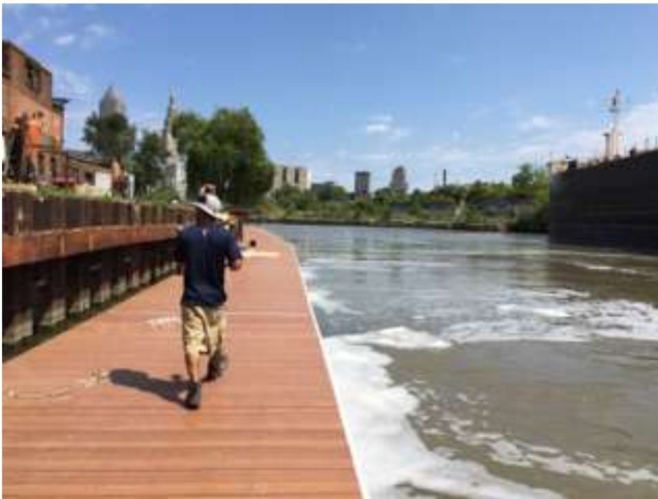
BoardSafe 50 Series Low Profile Docks being installed
