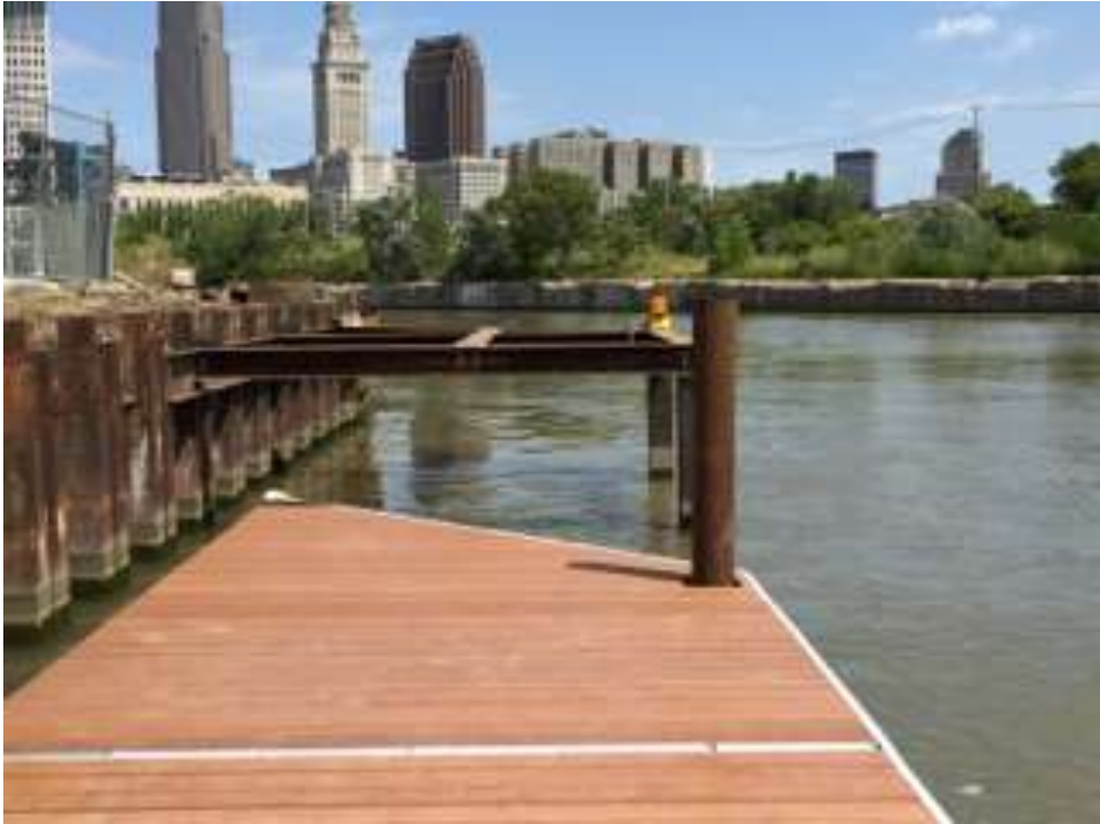
BoardSafe 50 Series Low Profile Docks being installed
