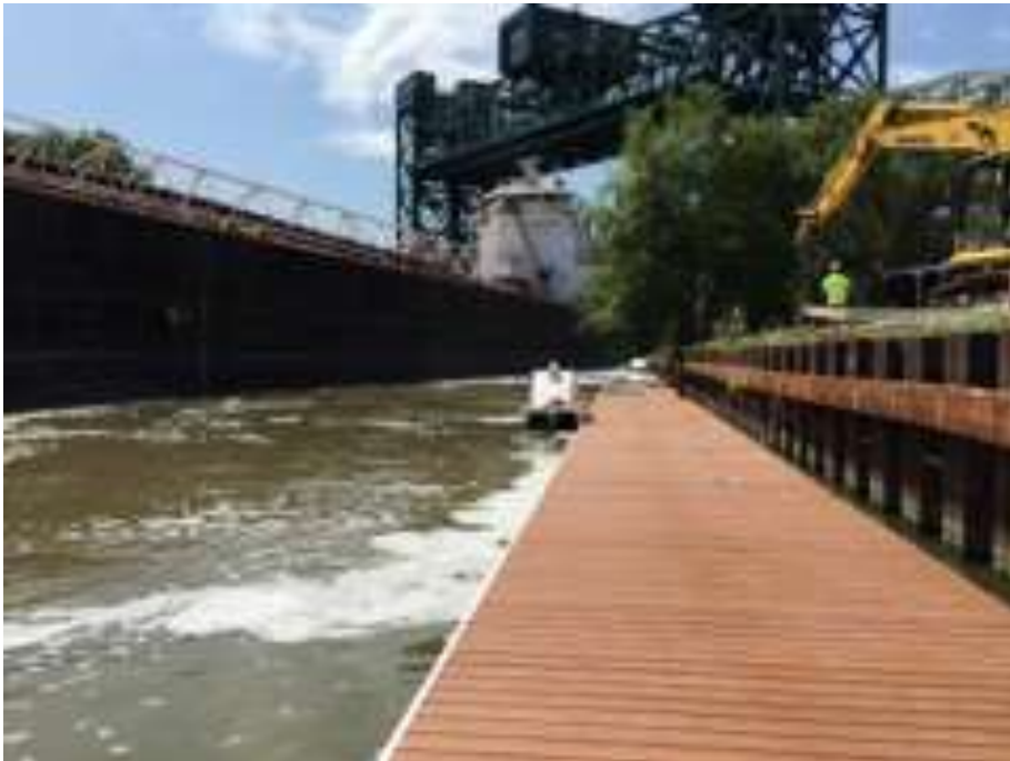
BoardSafe 50 Series Low Profile Docks being installed
